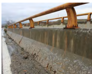
* Combined influence of ice, salt for de-icing and carbonization
