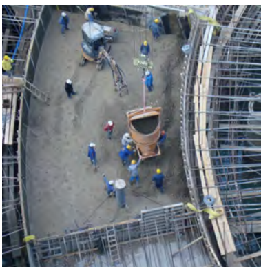
*Application of concrete with concrete bucket
