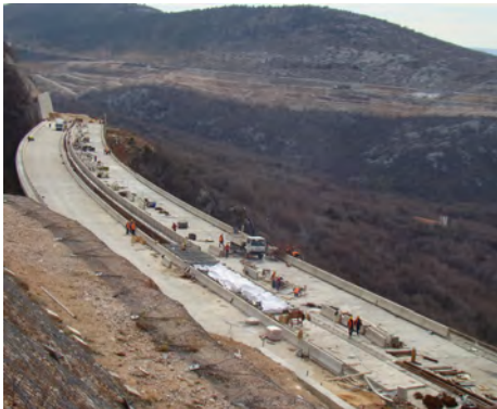
* Installation of waterproofing
