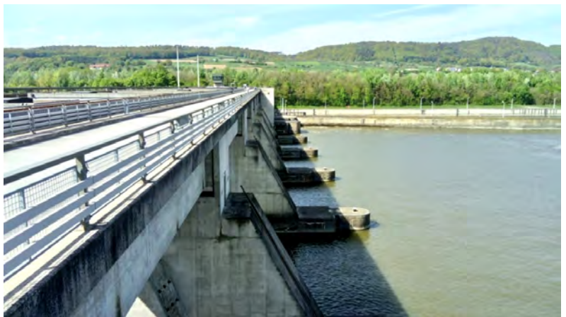
*Exposure of the structures to atmospheric and chemical influences
