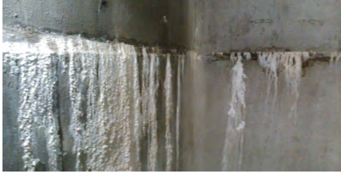
*Inadequate treatment of the construction joints
