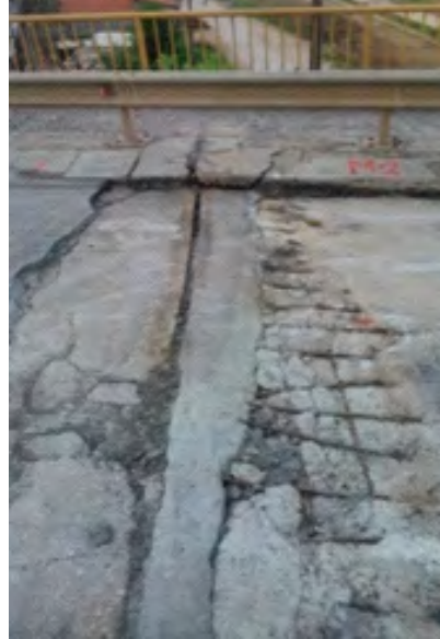
*Consequences of inadequate treatment of the expansion joints of bridge construction
