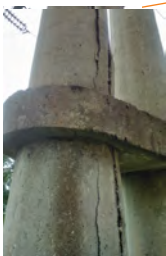
*Electric-chemical corrosion
