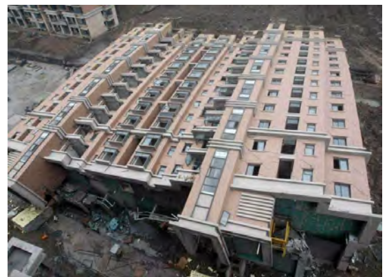
*Consequence of uneven consolidation of the foundations of the structure
