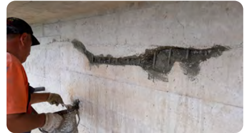
*Applying Reparatur Penetrat
