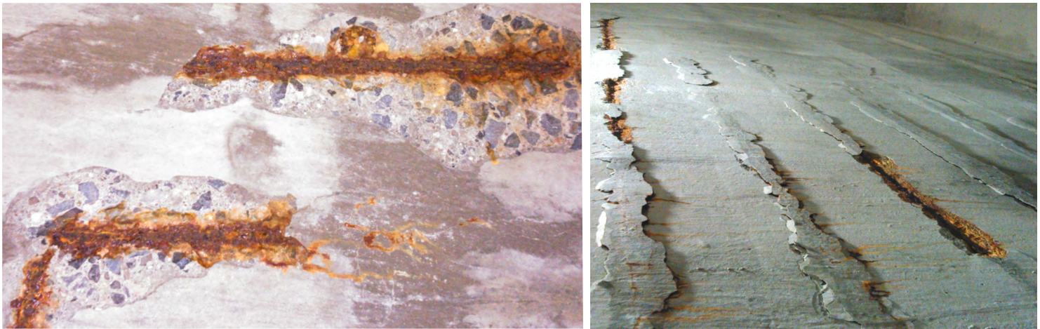
* Steel reinforcement corrosion, caused by concrete carbonation
