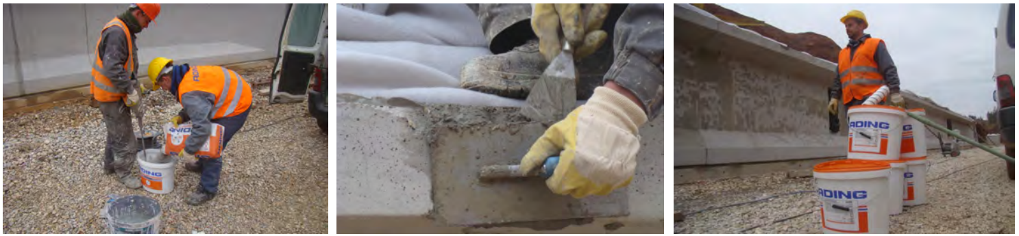
*Hand repaired concrete with Reparatur Malter F
