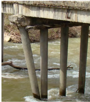
*Mechanical damage
