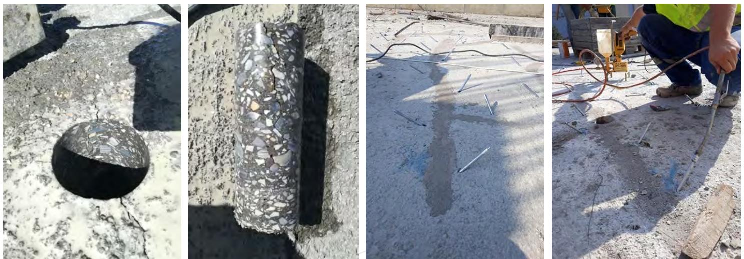
*Repair of crack in reinforced concrete slab, by injecting with Adingpoks I
