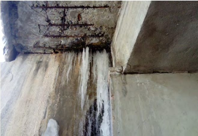
* Consequences of improper waterproofing
