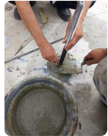
*Grouting anchors with Eksmal 1
