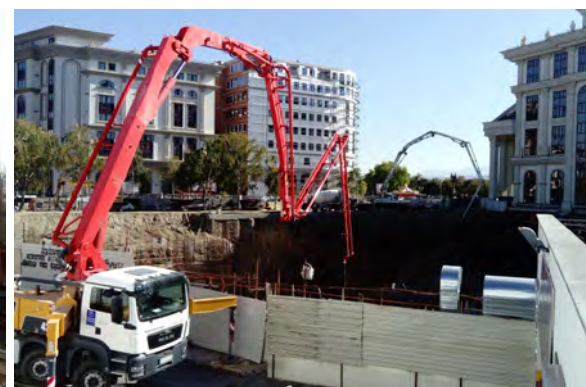
*Application of concrete with concrete pump
