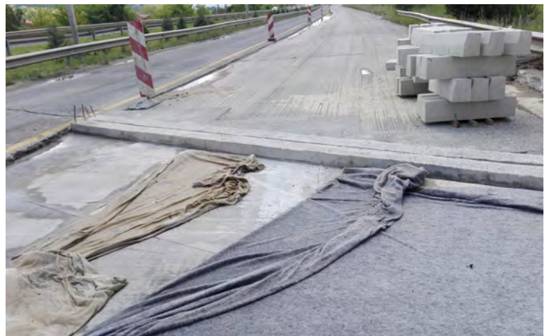
* Protection of fresh concrete by covering
