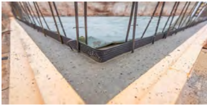
*Treatment of the construction joints
