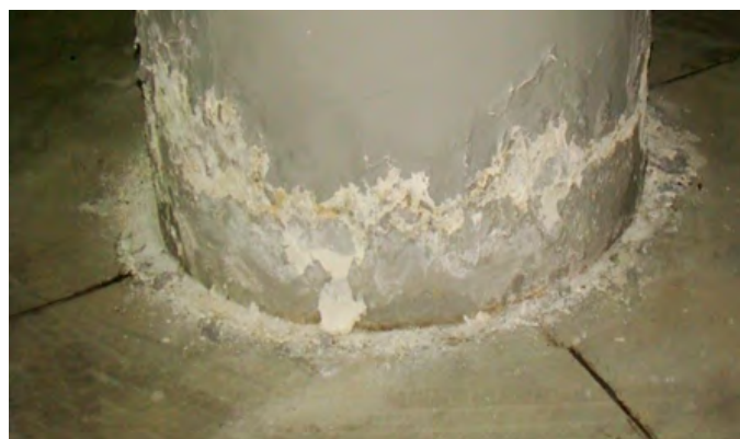
*Effect of capillary water absorption in concrete
