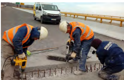
* Installation of expansion joints
