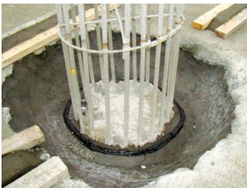
Penetration of reinforced concrete piles through foundation slab
