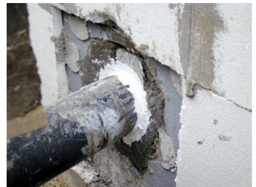
Penetration of pipe through an underground wall
