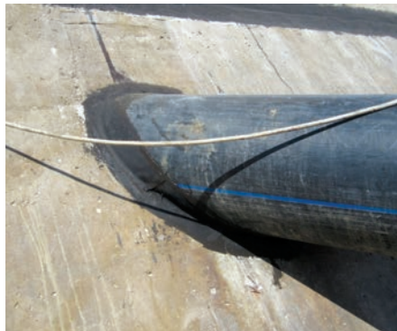
Penetration of pipe through the dam structure
