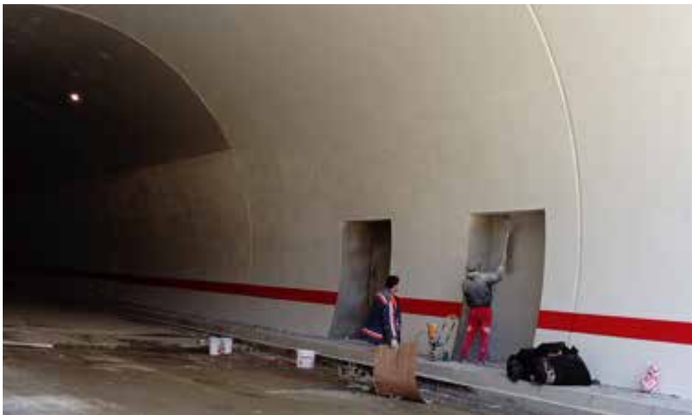
In situ examination of the properties of the protective coating AntikoroZin BB
