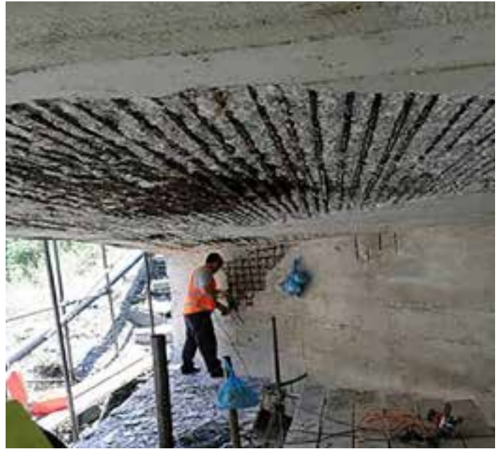
Corroded reinforcement as a consequence of concrete carbonation
