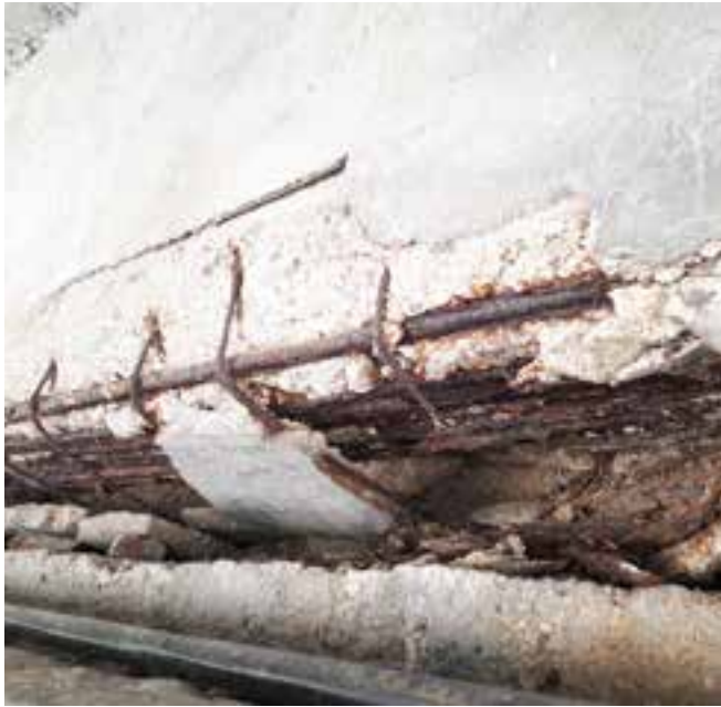
Corroded reinforcement as a consequence of concrete carbonation
